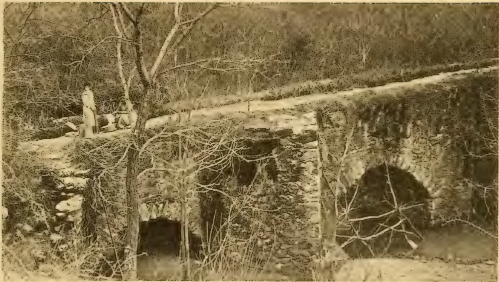
AQUEDUCT AT MISSION SAN JUAN.
